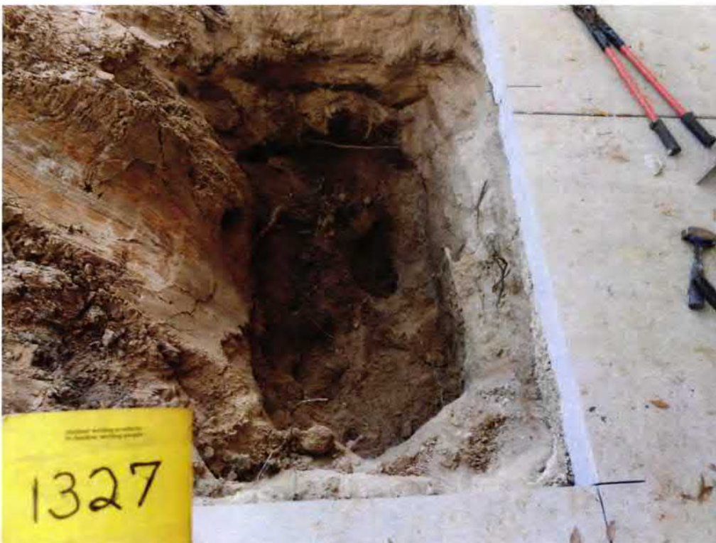
Picture 2: UST 1327Albatross being removed from the excavation.
